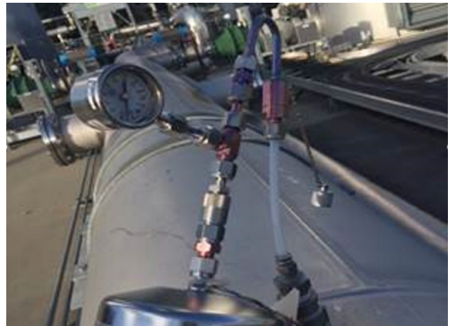
Tank Head Canister Sampling
